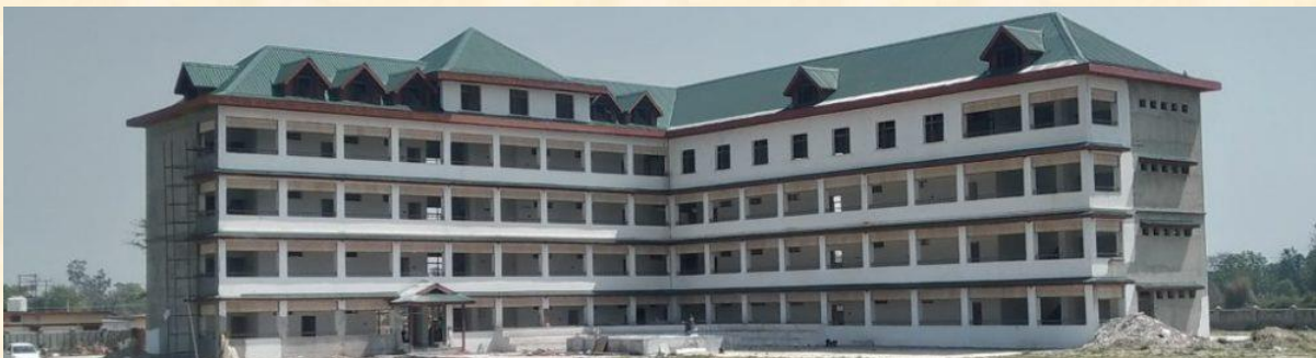
New College building.
